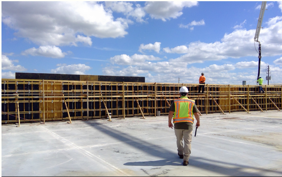
11 Million Gallon Plug Flow Digester Under Construction in Coopersville, MI
